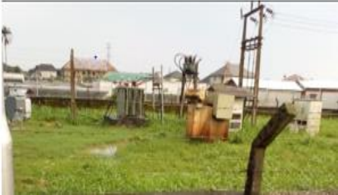
Plate 1: 2.5 MVA transformer and its accessories
