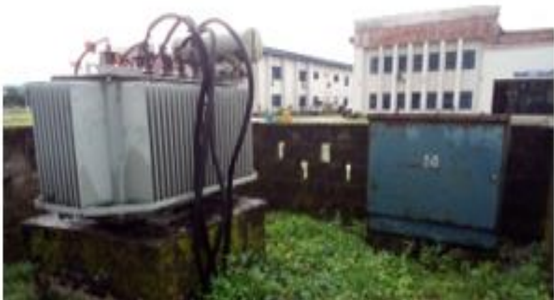
Plate 1: 2.5 MVA transformer and its accessories
